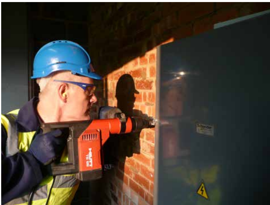
Figure 6.5 — Worker with a power tool held close to the body. In this situation exposure of the body and limbs will be similar and compliance with the low/high ALs will be limiting
